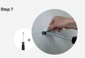
Place the concealed shelf supports over the fixings and screw lightly in place using the M6 bolts provided.
