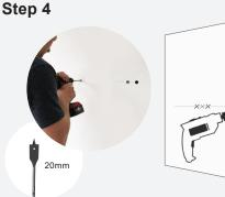
Using a 20mm spade bit, drill a hole on each of the outer marking to accommodate the Gripit fixings.
