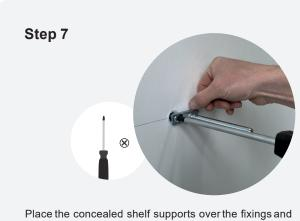
screw lightly in place using the M6 bolts provided.
